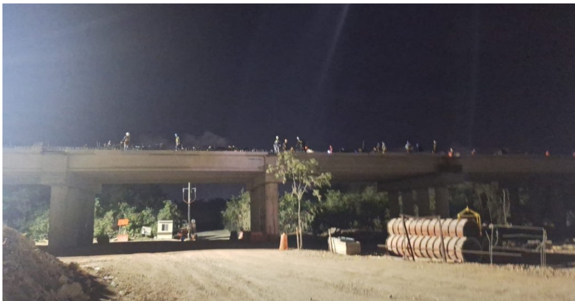
Night work on the elevated viaduct.
