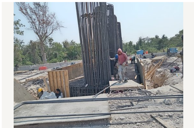
Formwork for foundation elements.
