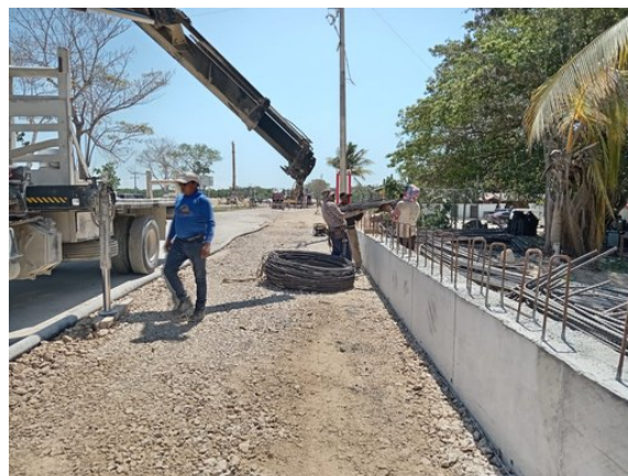
Boundary elements and associated works.
