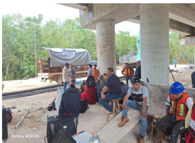
Construction personnel at the viaduct work front.
